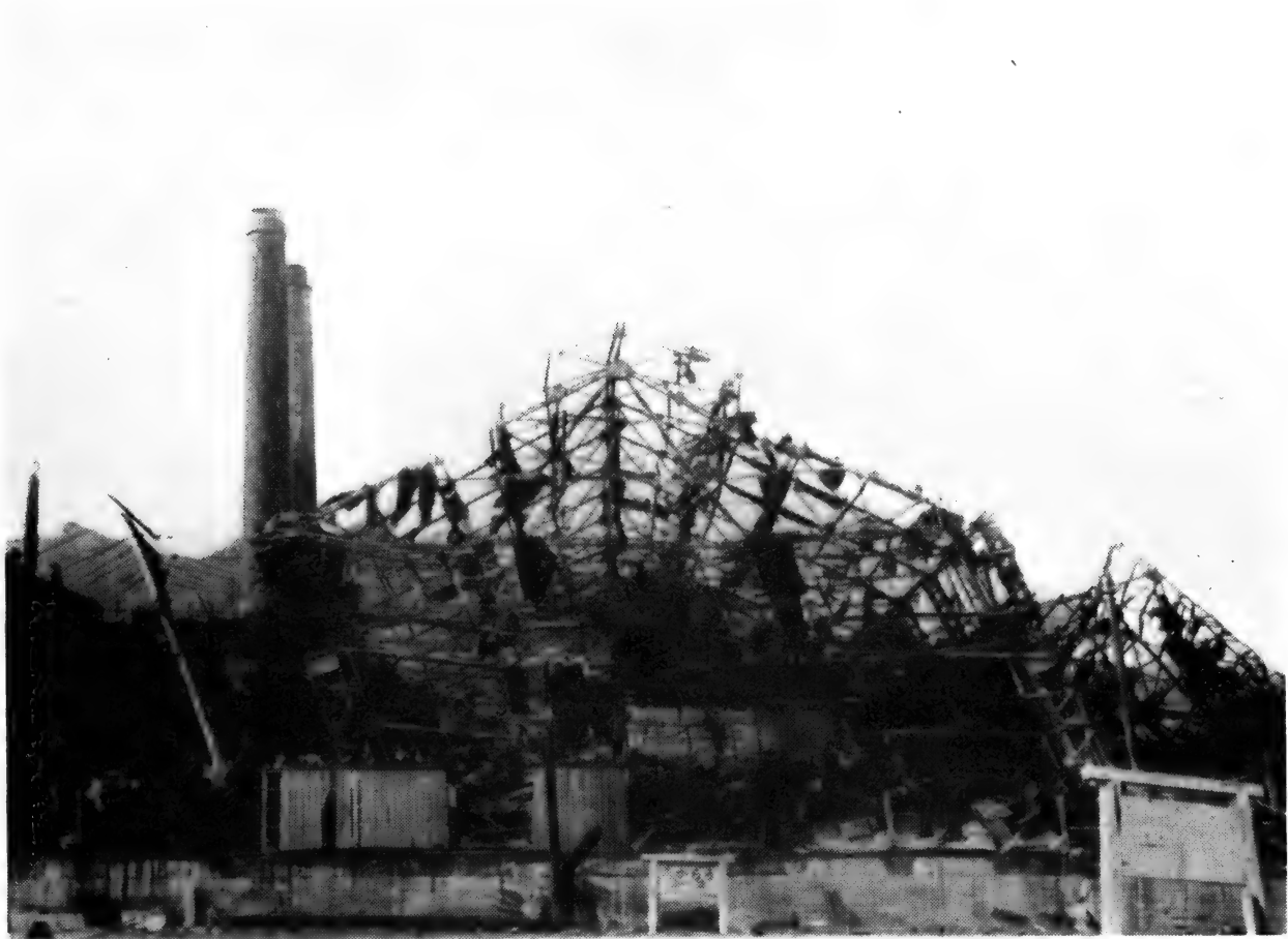
Photo No. 6. NAGASAKI. Mass distortion of steel framed shed buildings about half a mile from the centre of damage, which was to the right of the buildings in the photograph. It will be seen that the entire main frame is seriously distorted away from the explosion. See paragraphs 15, 22 and 32.
